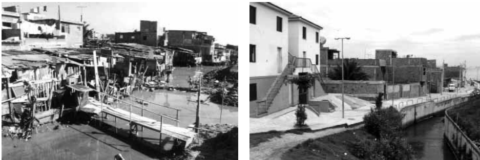
Figure 10 Photographs of before/completion of a slum upgrading project in Favela Barrios, Brazil
