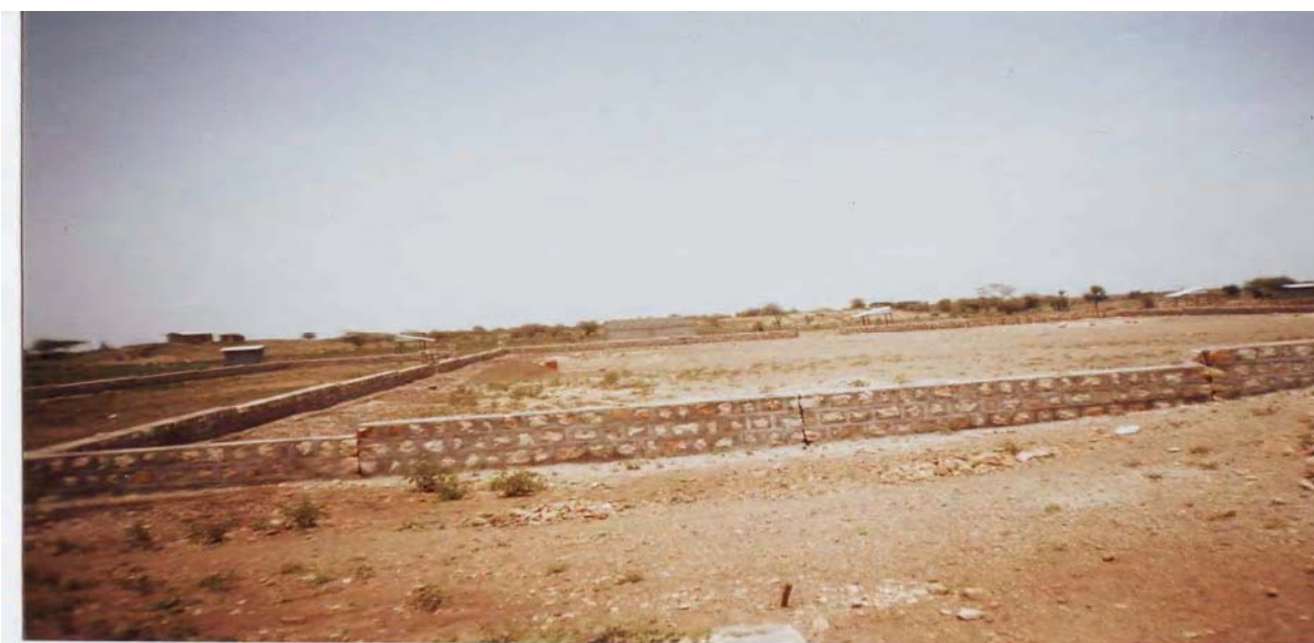
Figure 2: The new Chifra market under construction by ACDI/VOCA
