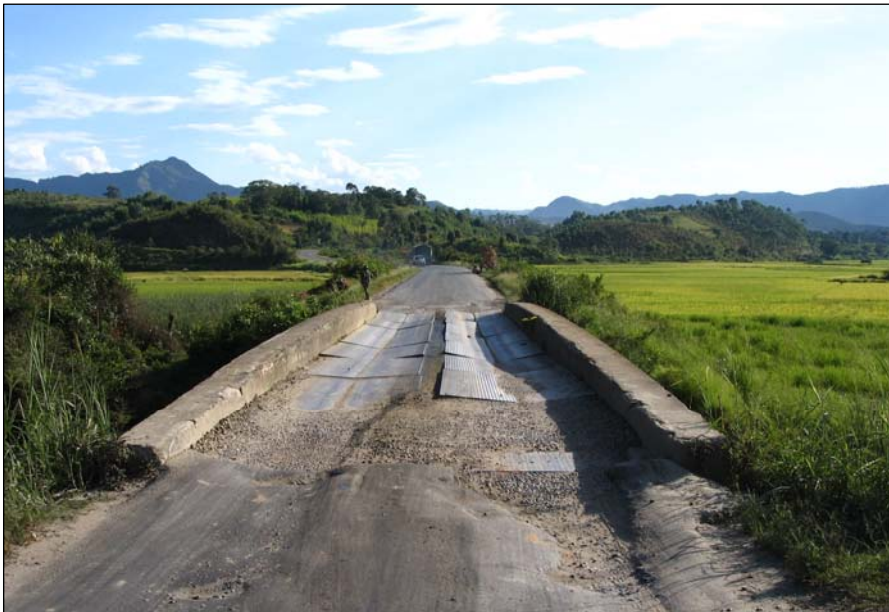
Figure 5.3: Bridge on Major Road between Antananarivo and Tamatave (Toamasina), the port
