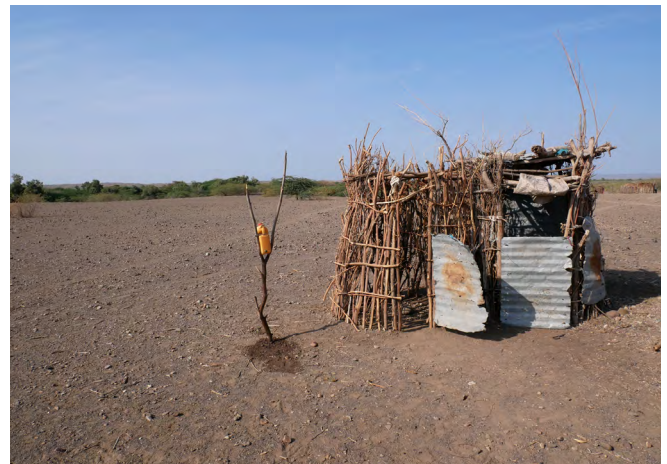
Latrine and shower shelter + hand-washing facility, Jeldi, Ethiopia. Photo credit: The Sanitation Learning Hub/Maria Gerth-Niculescu
