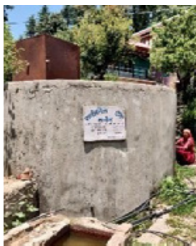
Plastic hoses attached to community tanks.
