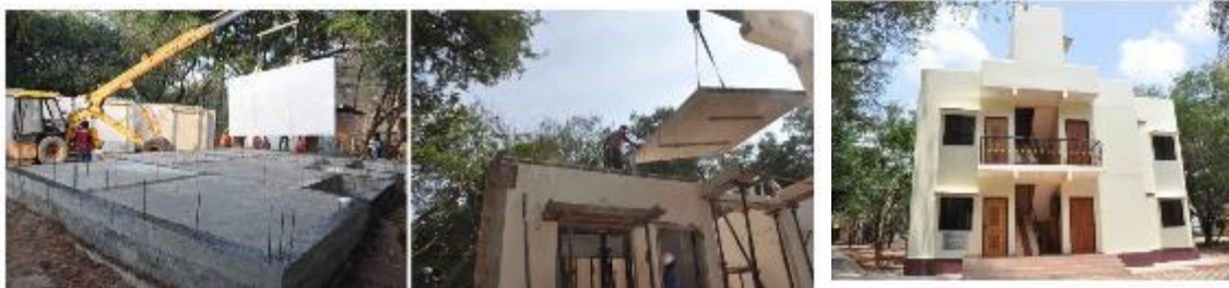
Figure 2 Construction of GFRG demo building
