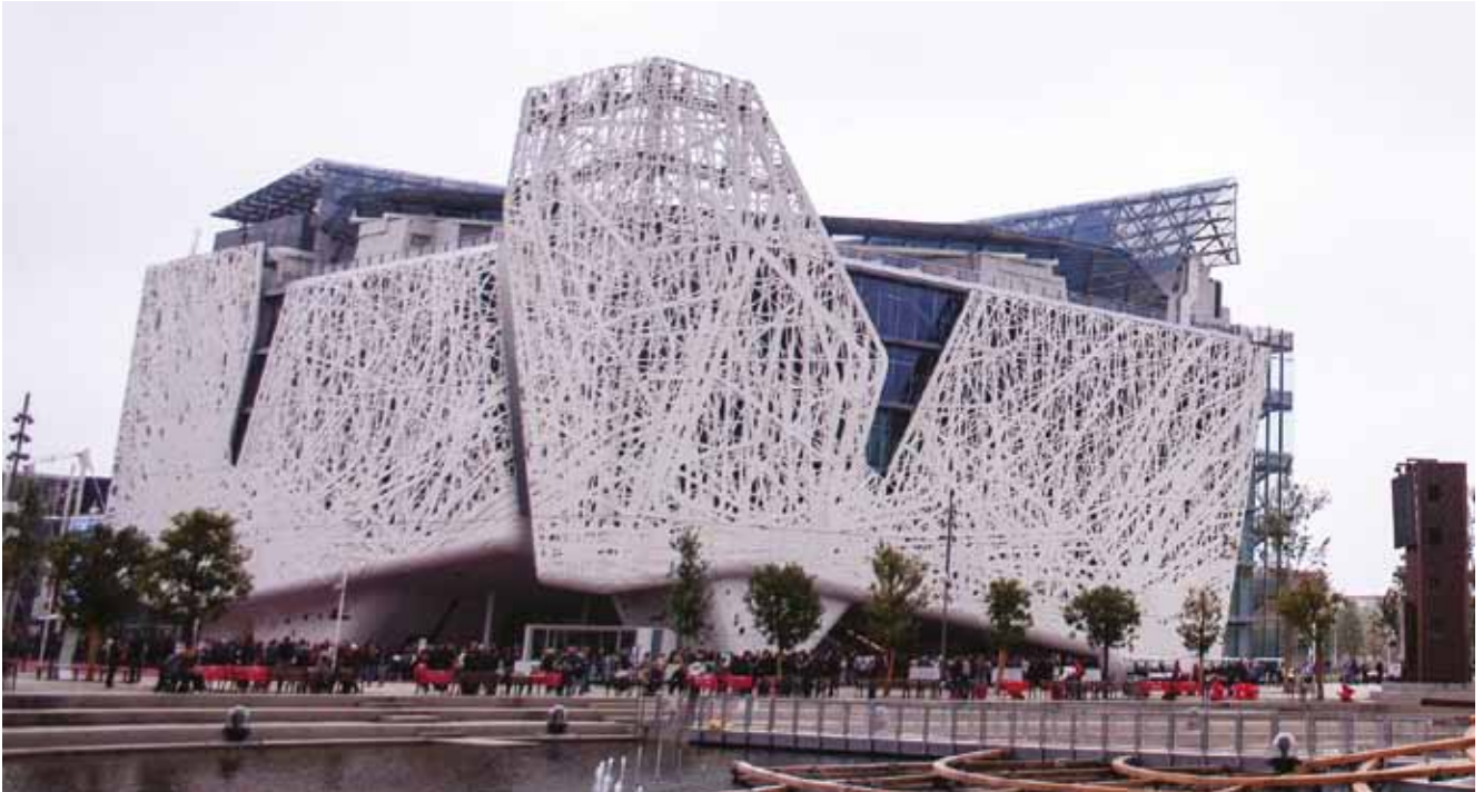
The Italian Pavilion in Milan has a facade that improves air quality by 'eating' smog when exposed to sunlight. Photo credit: Aumod on Pixabay, https://pixabay.com/en/milan-exhibition-architecture-1272520
