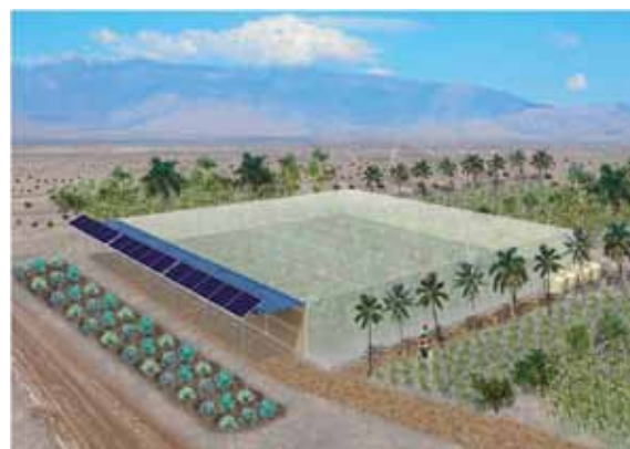
A Seawater Greenhouse in Somaliland aims to transform the hostile local environment into 'micro oases' to efficiently and effectively grow crops using solar desalination technology. Photo credit: Seawater Greenhouse, www.seawatergreenhouse.com/downloads/Somaliland%20Seawater%20Greenhouse%20Flyer.pdf
