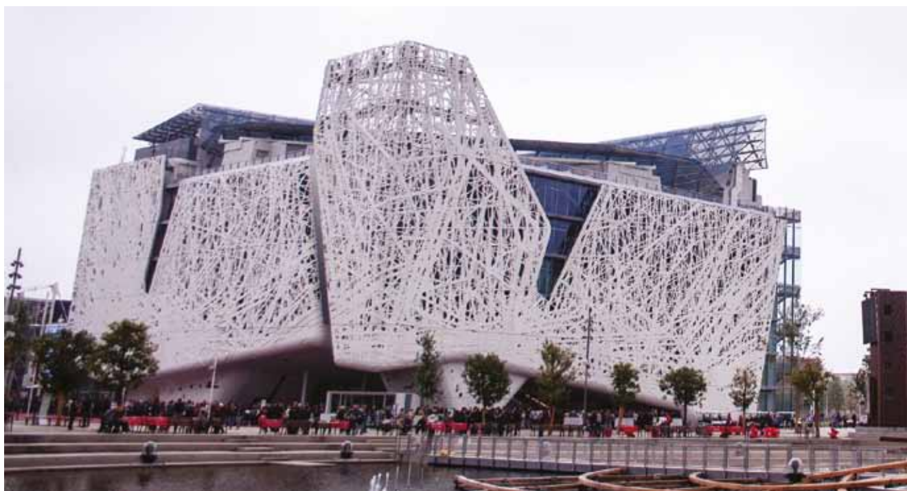
The Italian Pavilion in Milan has a facade that improves air quality by 'eating' smog when exposed to sunlight. Photo credit: Aumod on Pixabay, https://pixabay.com/en/milan-exhibition-architecture-1272520
