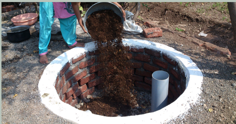
Tiger Toilet being installed, India. Credit: Claire Furlong.
