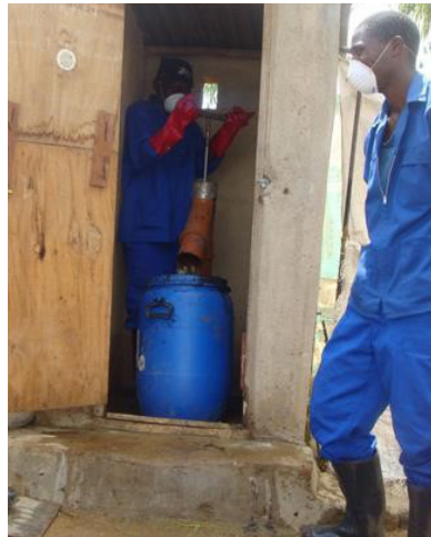
Gulper being used in Malawi. Credit: Joseph Magoya, Water for People.
