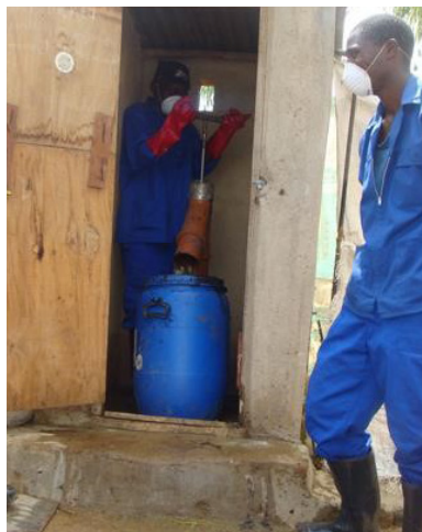
Bomba Gulper a ser usada no Malawi. Foto: Joseph Magoya, Water for People .
