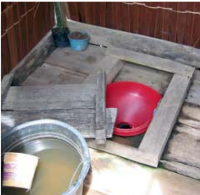
ABOVE A latrine constructed in South Sumatra, Indonesia. A woman used some household materials to construct a makeshift latrine in order to comply with the communities decision to go ODF, while her husband was away.
