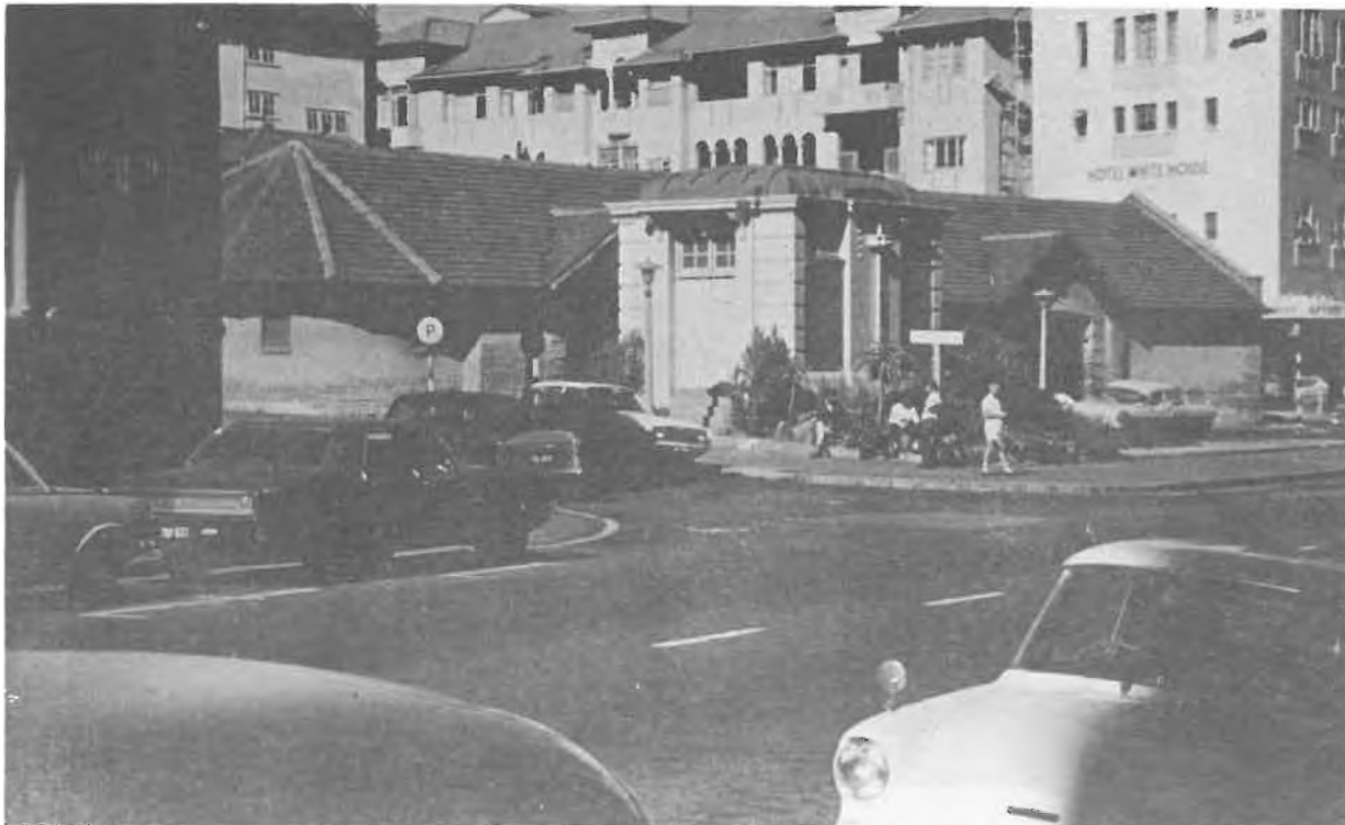
Plate 21 : Durban - Gillespie Street Transformer House
