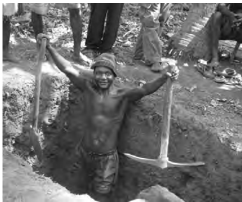
A young man starts digging his household latrine hole after triggering.
