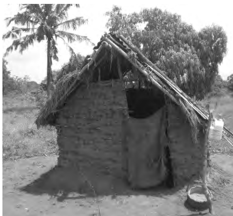
A simple pit latrine in Vitengeni, Kilifi District, Kenya.
