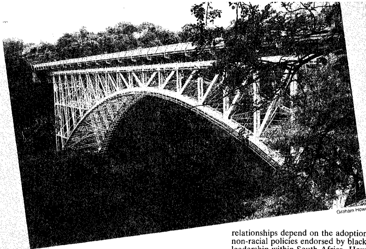
The Victoria Falls rail bridge connecting Zimbabwe and Zambia. Most of the frontline states' export goods carried over this bridge are eventually destined for export through South African ports.
