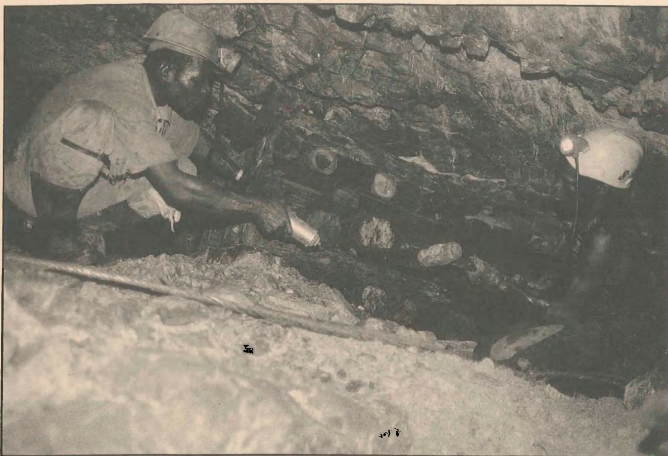
Western Deep Levels Mine, Carletonville. Safety hazards and the high underground fatality rate in the South African mining industry have become controversial labour issues in the 1980s.
