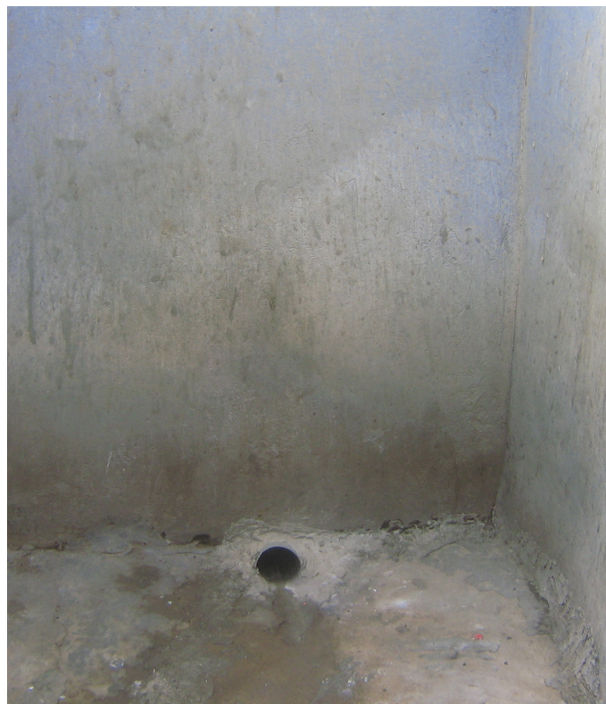
Figure 3: Bathhouse in Kumasi, with drainage connection
