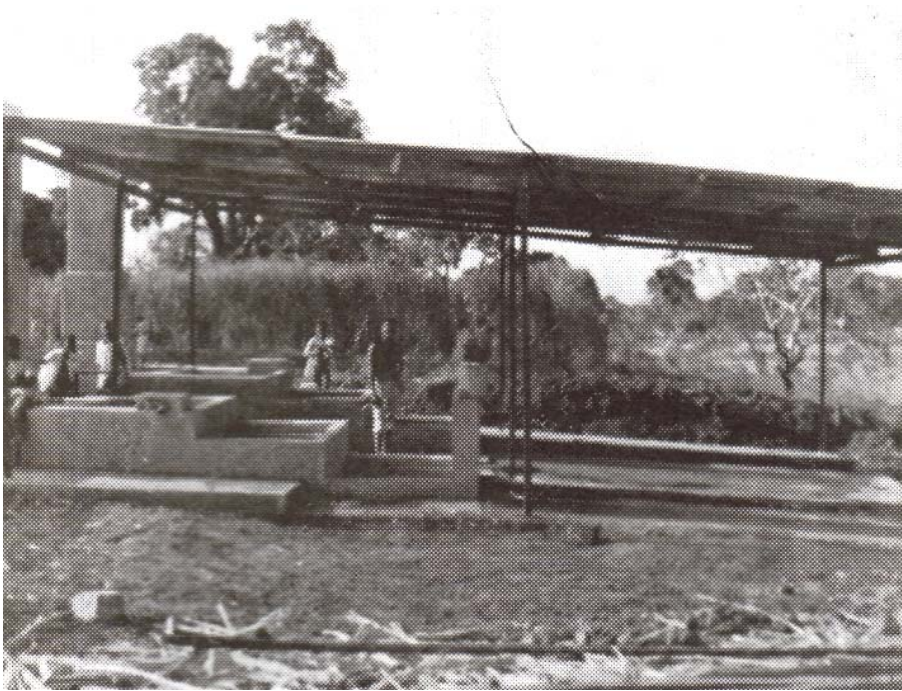
Figure A2: Photograph of Evaporators
