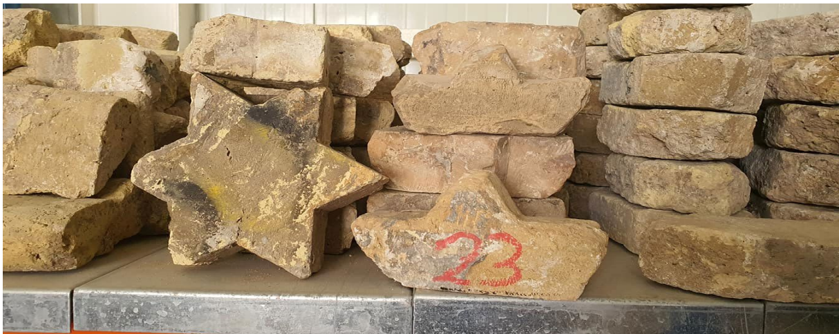
Figure 8. Numbering the collected blocks of Al-Nouri Mosque
