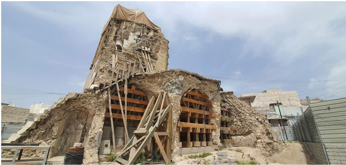
Figure 6. Al-Hadba Minaret surrounded by timber structures
