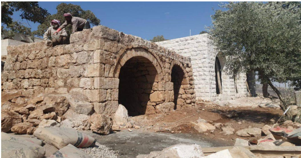
Figure 10. Replacing old blocks with new ones outside the shrine
