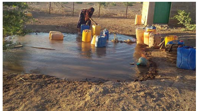
Figure 12: Woman collecting water from a broken pipe. Photo: Mahisa
