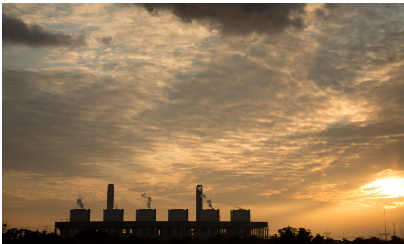
Medupi Power Station in Lephale, Limpopo. Photographer: The Dollie House. © IDS.
