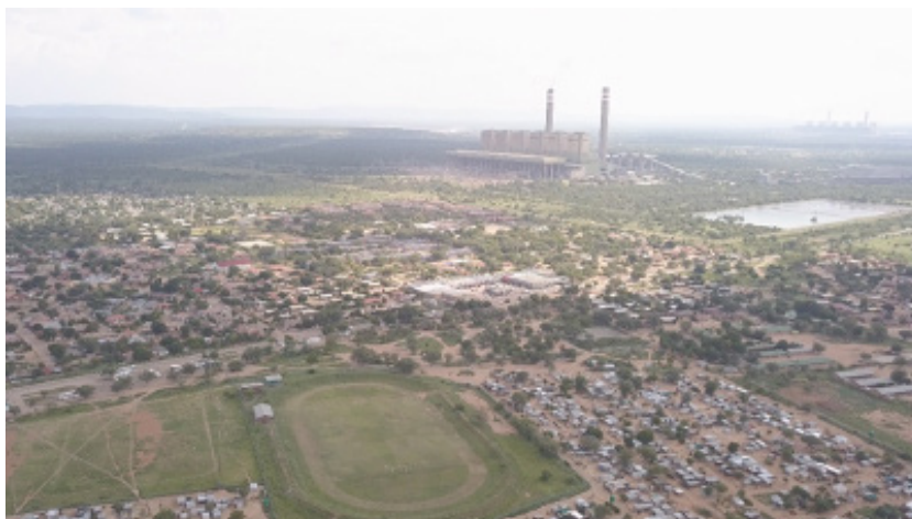
Aerial view of Lephale Town with the Matimba and Medupi power stations in the background.
