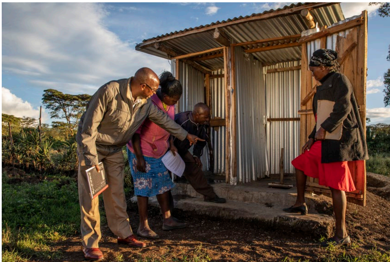
A latrine in Hells Gate community, Nakuru county. The owners, John and Virginia Njogu built the toilet after their community was triggered. Solomon Ndungu a CLTS coordinator and Ekrah Wairimu a local VSC make a follow visit to inspect the latrine and hand washing station along with a Peter Murugu a PHO (Credit: Jason Florio)
