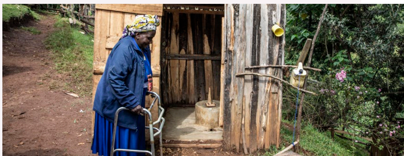
Christine Silate, a disabled (amputee) women in Botoret village. The VSC constructed a toilet for Christine with a raised seating platform specifically for her challenges. (Credit: Jason Florio)
