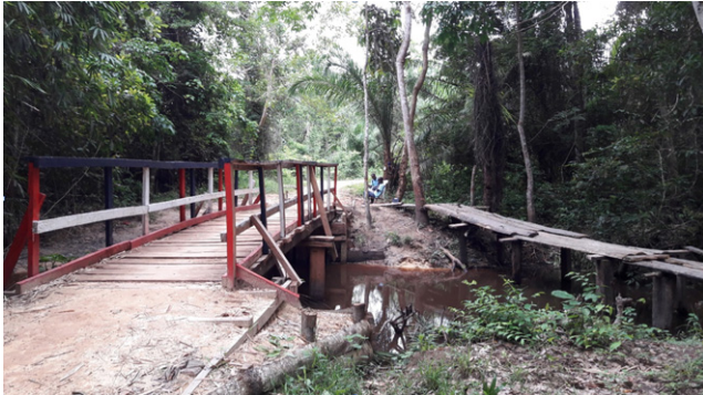
Figure 5. Newly constructed 'engineered timber bridge' (left) and old locally constructed bridge (right)
