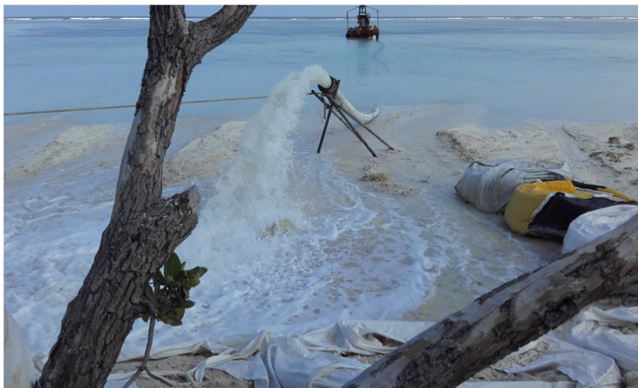
Fig. 2. Sand pumping for beach renovation.
