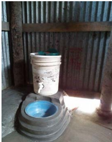
Used paint container with tap and installed inside the kitchen along with plastic bowl for basin
