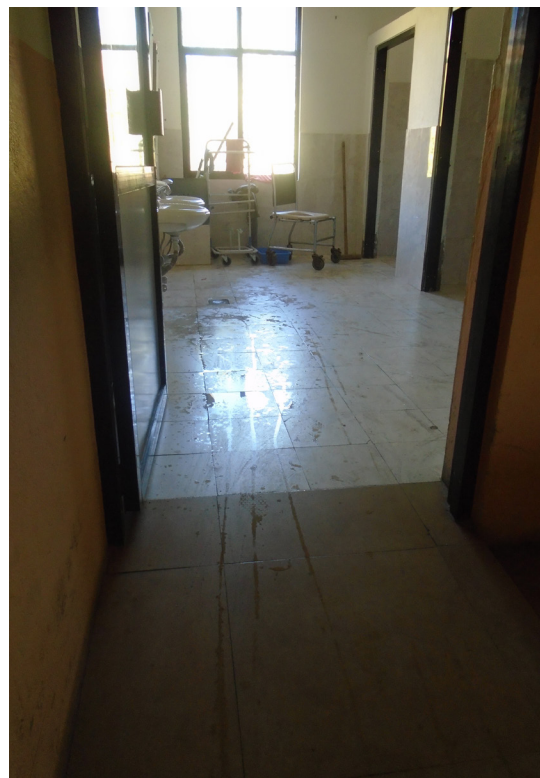
Figure 10: 'During period one should be careful using bathroom. Our legs might already feel weak (lulo) so we might fall down and meet an accident. Here the toilets are made for everyone to use but if it was to be built at home for crutches user, it is to be made in a way that it is not slippery. Marble should not be used as it is slippery.' (Photo: Babita Thapa, Nepal)
