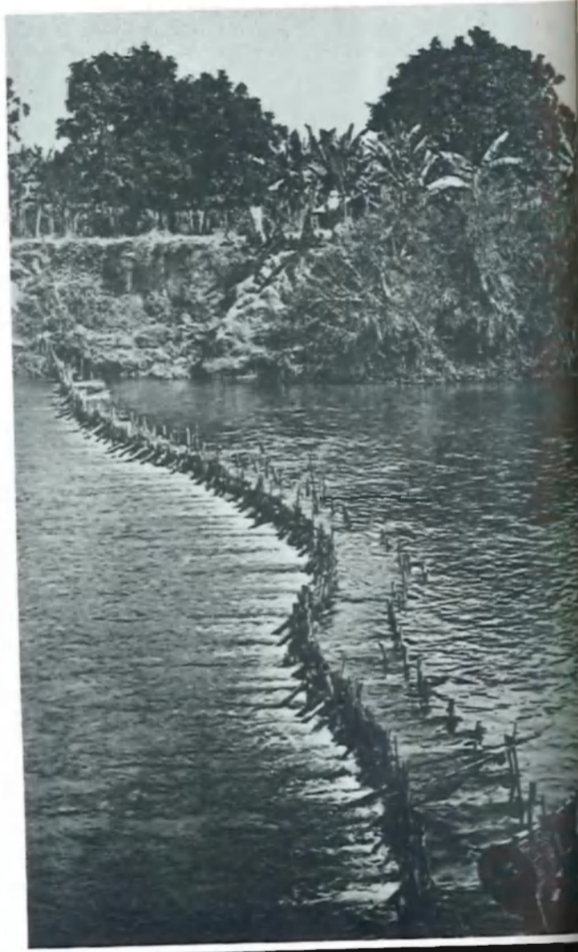
Fish dam on the Kiwira River
