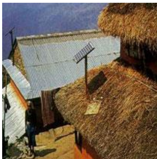
Figure 4.2: Solar Home System
