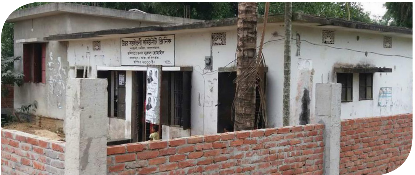
The security of Uttar Baraitali Community Clinic was always a concern. Post CSC implementation, through collective action of the CSG, CG and local government, a boundary wall was built around the premises.
