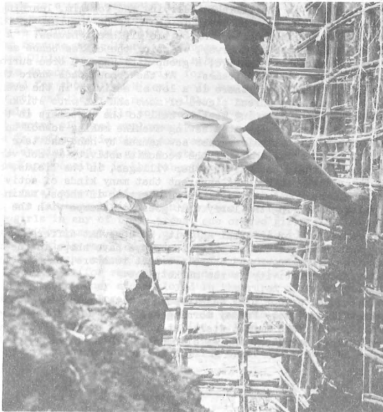
HOUSEBUILDING IN KALUNGA
