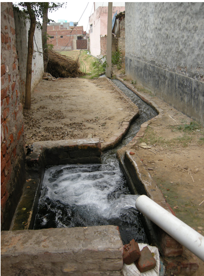
Drainage channels in Karhera
