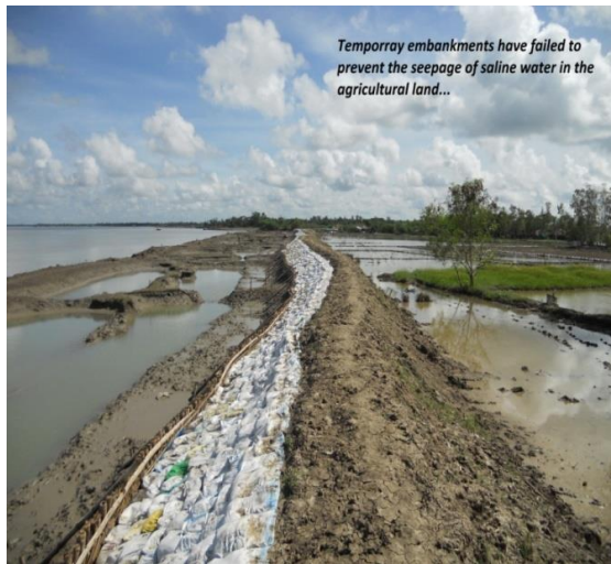
Figure 7.2: Temporary Embankments
