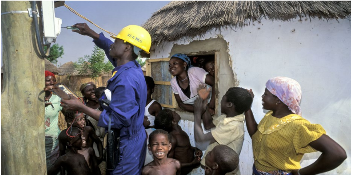
◀ Ghana. Electricity installation engineer in a rural community.
