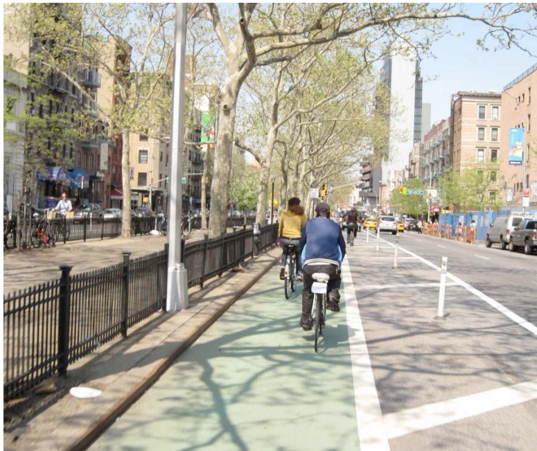
Figure 14: This cycle track along Allen Street in Manhattan provides safe, convenient, and pleasant cycling, completely separated from motor vehicle traffic. (Source: Nicholas Klein)
