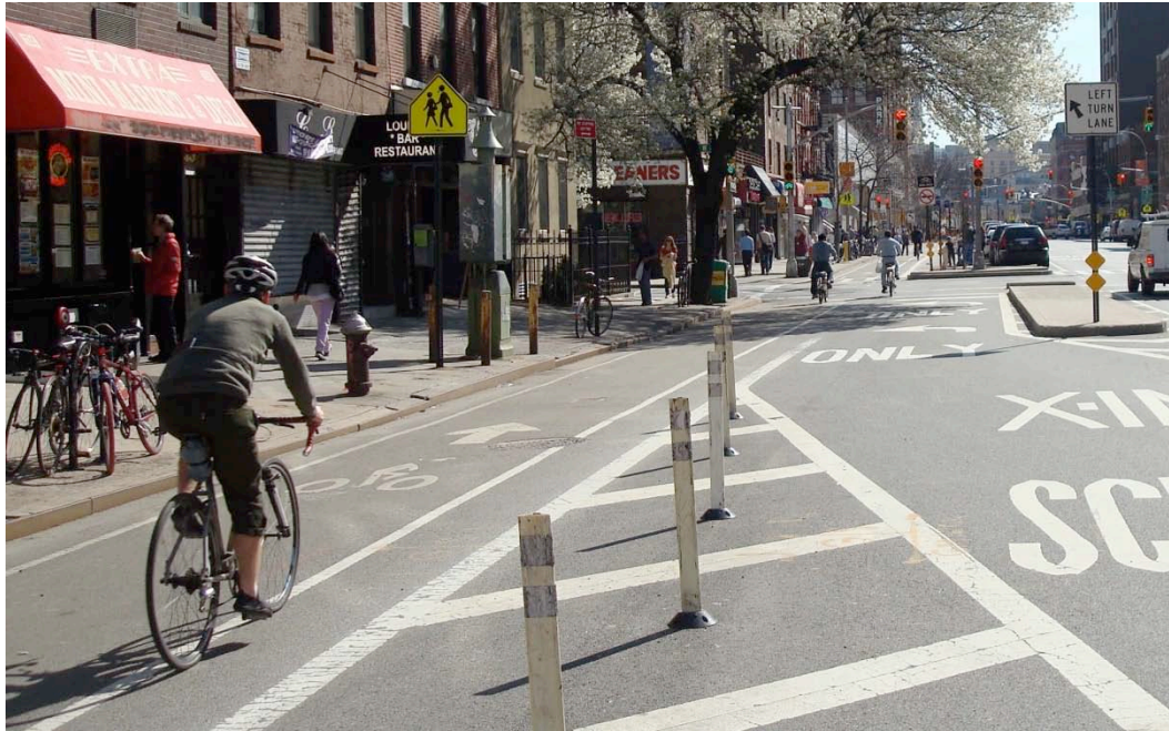
Figure 15: The 9 th Avenue cycle track in Manhattan is designed to minimize conflicts with left-turning cars, both through lane design and traffic signals. (Source: Lewis Thorwaldson)
