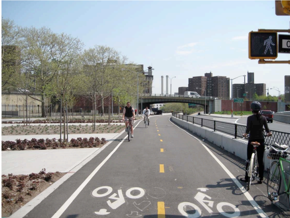
Figure 17: The Sands Street cycle track in Brooklyn, near the Manhattan Bridge, is bi-directional and offers complete separation from motor vehicle traffic. (Source: Nicholas Klein)
