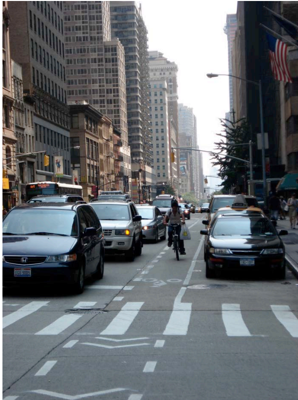
Figure 24: Many bike lanes in New York are too narrow and subject cyclists to the dooring hazard because of the proximity to parked cars, as here on 6 th Avenue in Manhattan. (Source: Ralph Buehler)
