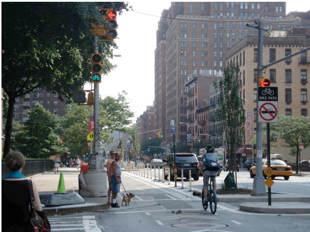
Figure 16: Special traffic signals along the 9 th Avenue cycle track protect cyclists from left-turning motor vehicles, while pedestrian crossings are facilitated by median islands. (Source: Ralph Buehler)
