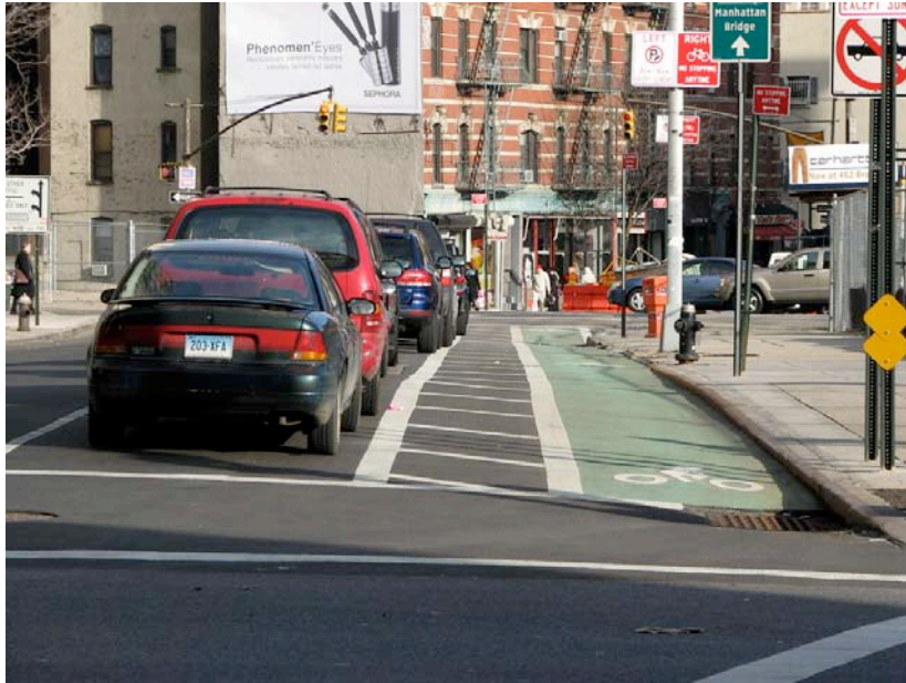
Figure 20: The diagonally striped buffer zone on the Grand Street bike path enhances cyclist safety by increasing the distance of motor vehicles from cyclists, but it provides no physical barriers. (Source: Nicholas Klein)
