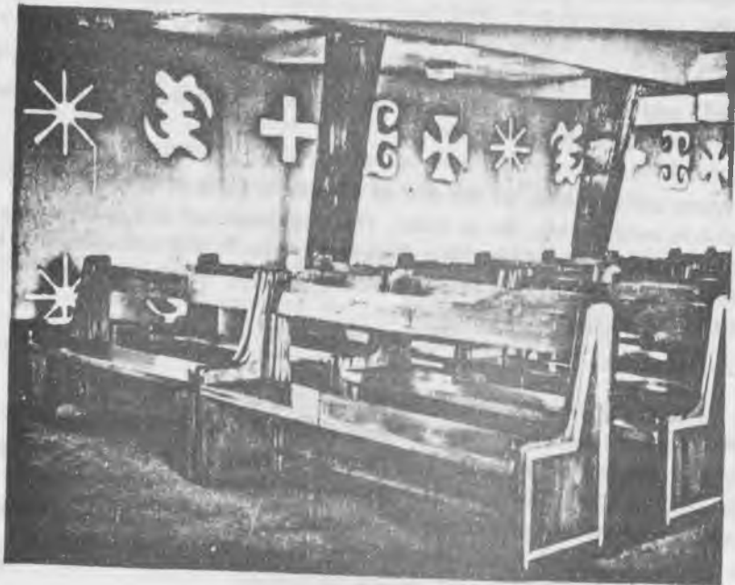
2. A side of the wall from inside the Church. The motifs serve as ventilations.
