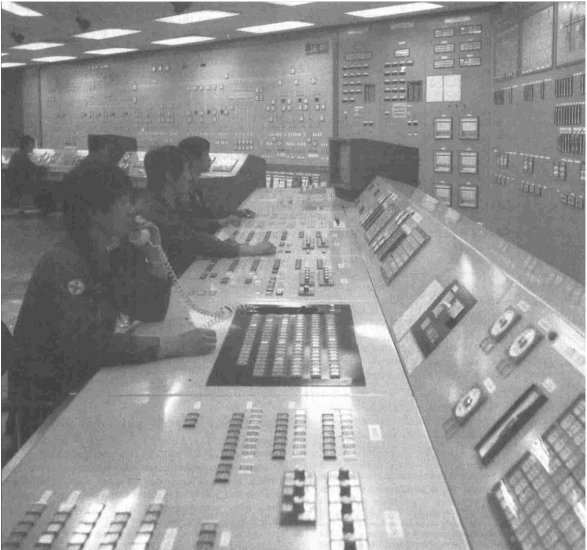
Energy centre at Pohang Iron and Steel Co Ltd, equipped with remote control system for power receiving and distributing stations and gas and heavy oil facilities.
