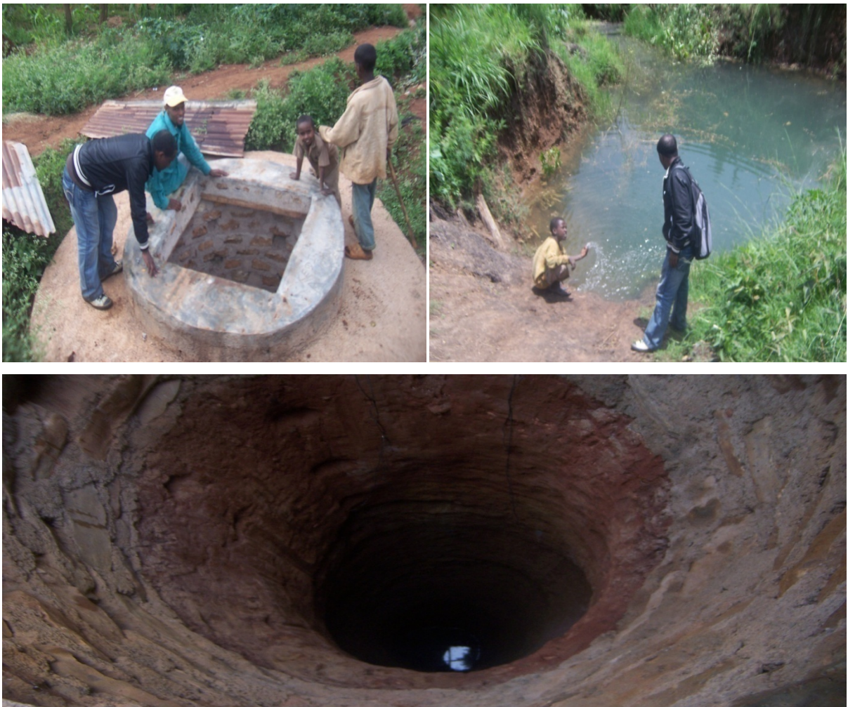
Picture 4.1: One of well prepared groundwater wells (Upper left) and the most commonly used type of groundwater well (upper right) in Damota and the most common type of borehole in Melka Gemechu (bottom).
