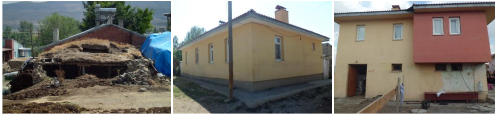
Figure 6 A picture of a house collapsed; the samples of single-storey and two-storey buildings from the implementations completed by the end of 2004 (D G Yilmaz 2013).
