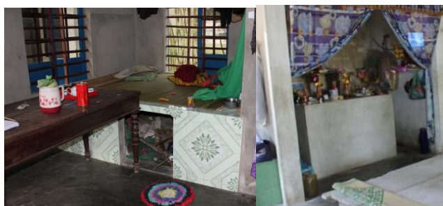
Figure 6 RC bed (left) and RC altar (right) were found in all surveyed houses
