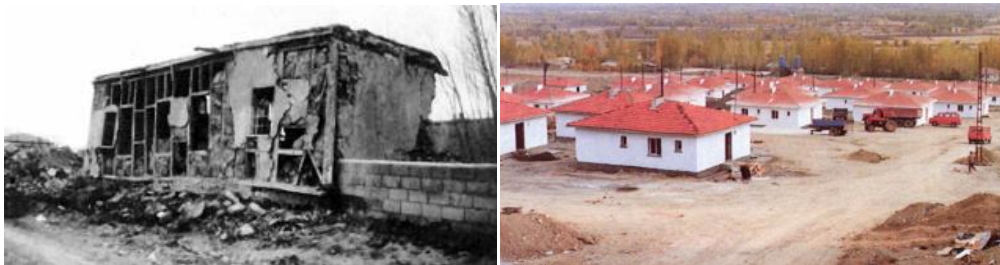
Figure 3 A picture of a heavily damaged adobe infill-wooden frame house from the village of Altınbasak (Williams et al. 1992); the reconstruction phase in the same village (The Ministry of Settlement and Public Works of Turkey 1993).
